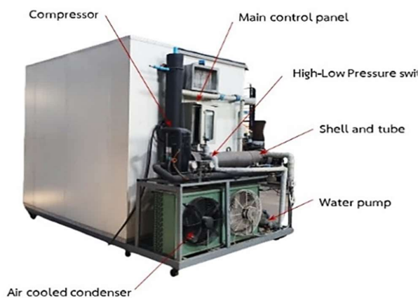
Figure 7 Hydro heat pump system component.
