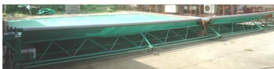
Figure 2 Frame and Cover Assembly.
