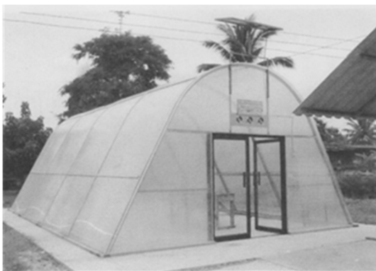
Figure 1 Solar greenhouse dryer parabola shape.
