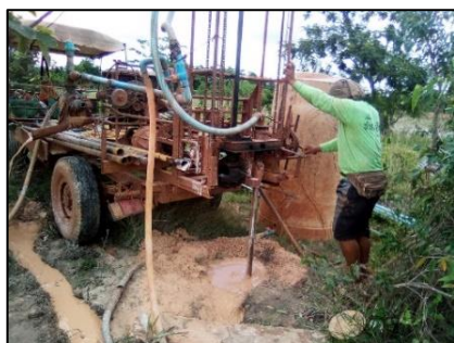
Figure 3 Water well being drilled for groundwater data
