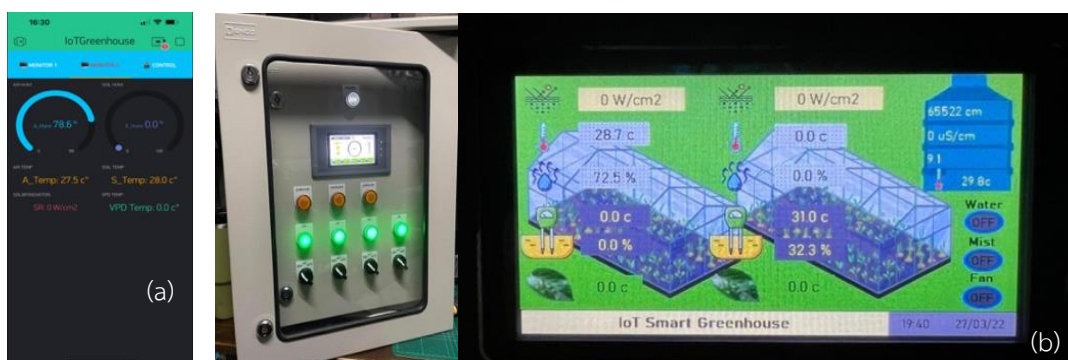
Figure 4 Monitoring IoT environmental sensors monitor using Blynk application (a) IoT sensors status show on HMI displayed(b)
