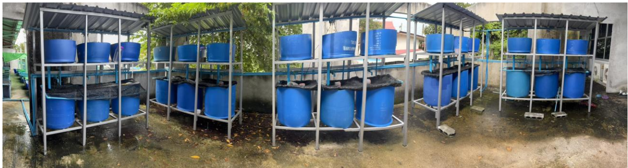
1a. Small-scale Recirculating Aquaculture System (RAS) layout showing stacked filter and rearing barrels constructed from blue plastic drums.
