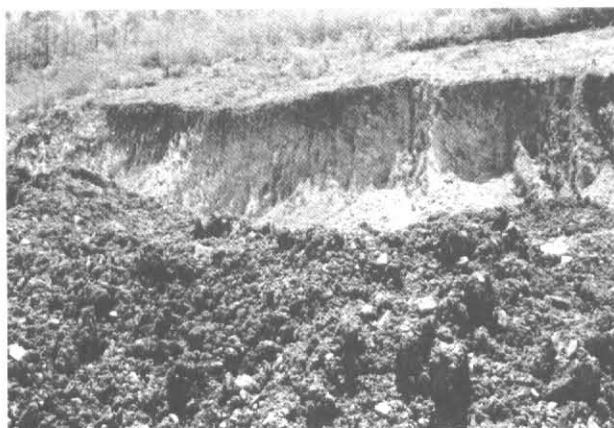
Figure 1 Test trench excavating at the toe of the mild hill side.
