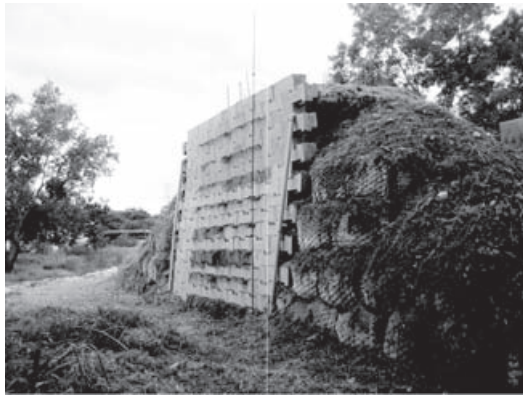
Figure 3 Completed full scale test embankment Construction.
