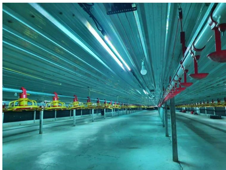
Figure 2 Inside broiler barn with installed dimmable light system.
