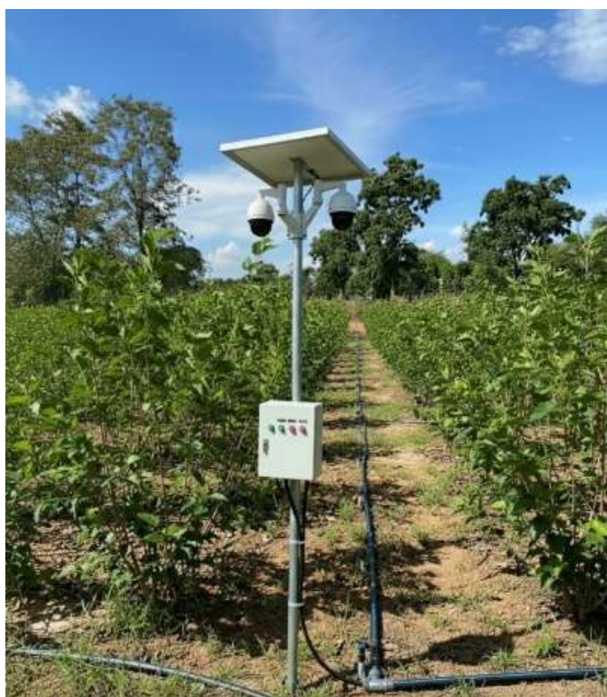
Figure 4 Installation of smart farm control system on a mulberry farm
