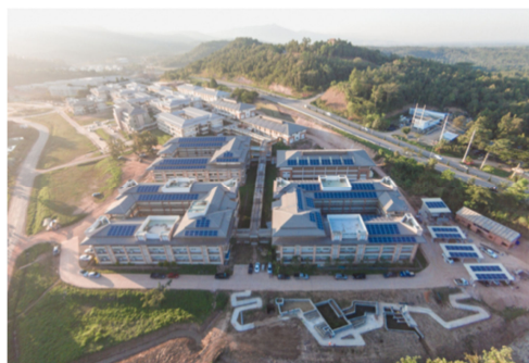
Figure 2 The installation of photovoltaic cell system on the smart grid networks in the University of Phayao.
