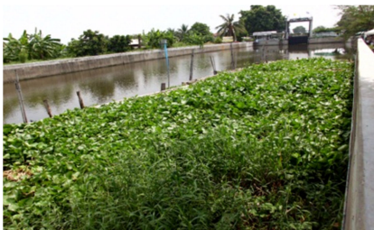
Figure 2 General condition of Klong Muang canal.
