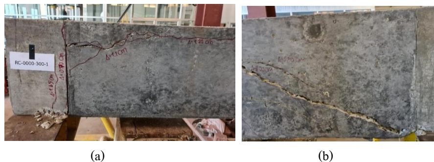
Figure 10 Failure of the beam specimen Group 2:
