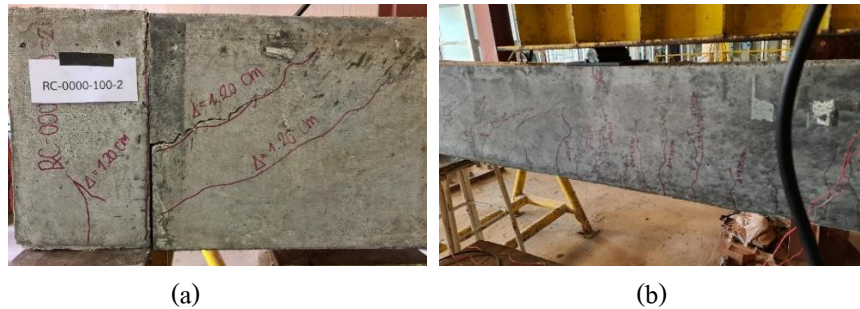
Figure 9 Failure of the beam specimen Group 1:
