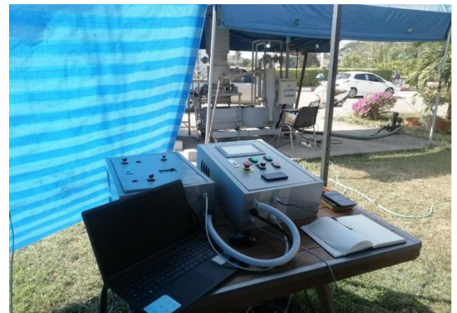
Figure 6 Installation of automatic control cabinet to V-Hearth gasifier
