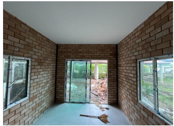
Figure 12 Color of interlocking blocks with rubber wood ash admixture inside a house.
