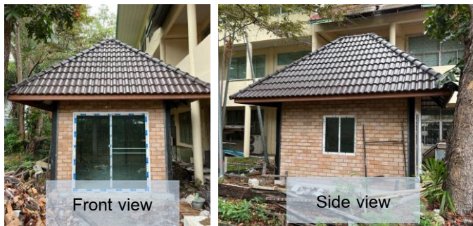
Figure 10 House built with interlocking blocks containing para-wood ash.
