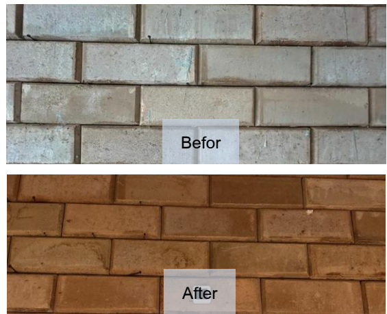
Figure 13 Changes in the surface color of interlocking blocks with rubber wood ash admixture on the exterior of a house.
