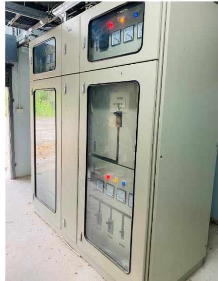
Figure 1 The Main Distribution Board (MDB) used for analyzing the relationship between features influencing the occurrence of unbalanced current.
