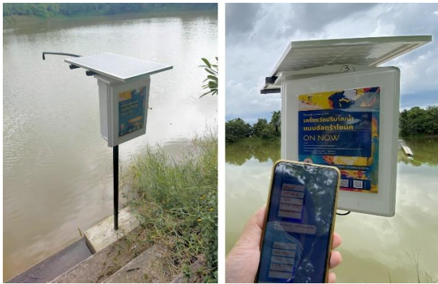
Figure 5 Field installation results.
