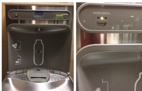
Figure 4 Drinking water machine with the filtration status
