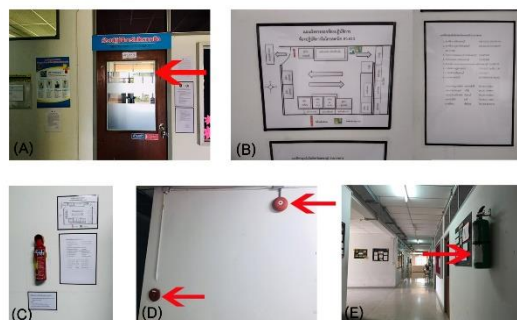
Figure 11. (A) Vision panel door, (B) Layout showing important information, (C) Portable foam fire extinguisher, (D) External hand fire alarm system and (E) Install fire extinguisher at less than 150 cm height from floor to discharge lever (after the implementation)
