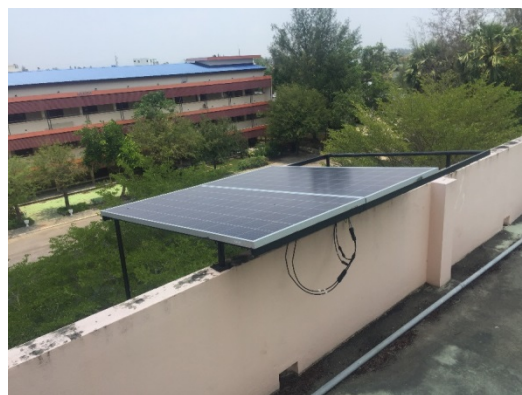
Figure 3. Installing solar cell on the roof
