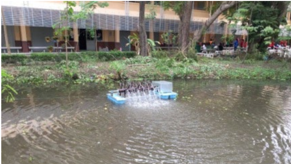
Figure 5. Equipment installation of oxygen in wastewater wells
