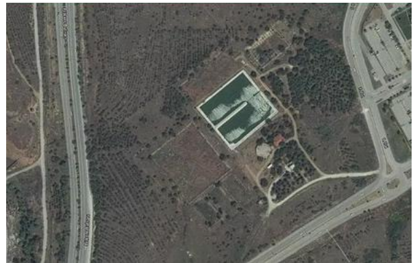
Fig. 12 Aerial view of the water recycling plant serving METU
