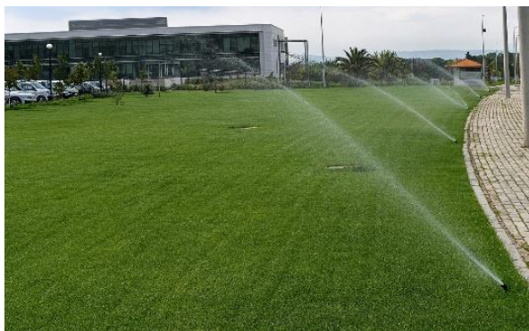
Fig. 13 Sprinkler system using recycled water for irrigation on METU's campus grounds
