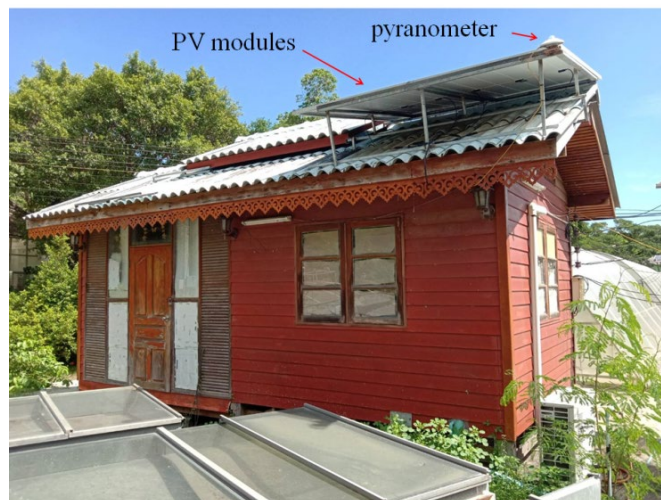
Figure 2. The hut for placing the modified refrigeration system
