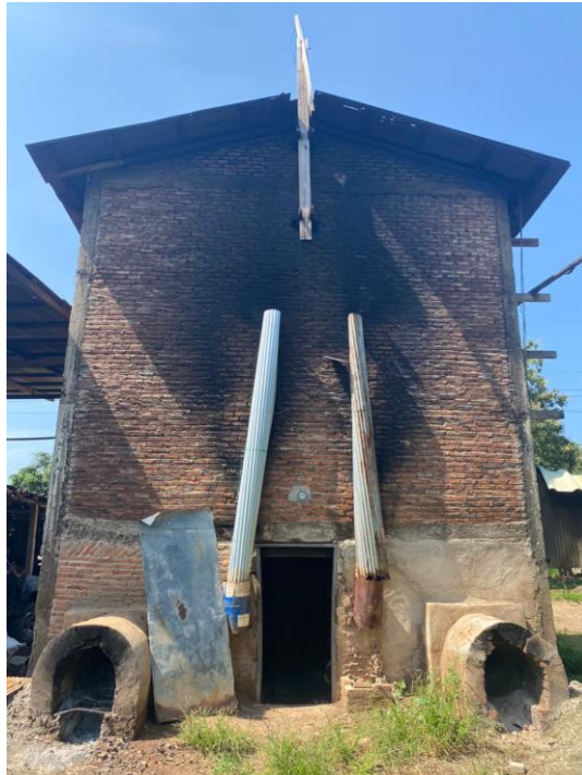
Figure 1 Direct heating kiln used to dry the pizza trays
