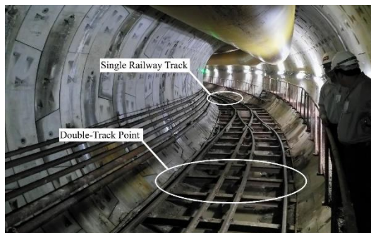
Fig. 3. Single railway track and double-track point
