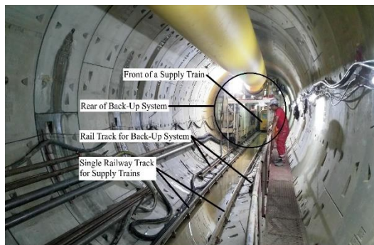
Fig. 2. Rail tracks for supply trains and back-up system
