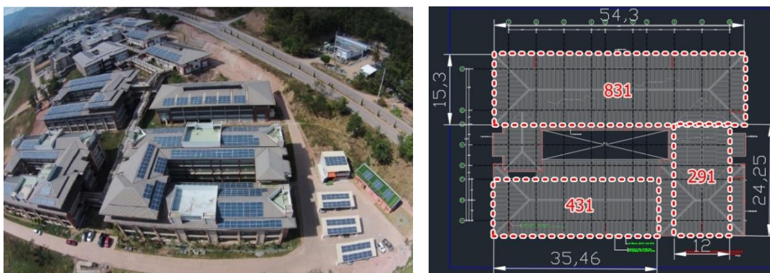
Figure 3 An installation of solar panels of the smart grid UP system and the roof area of the B3 building
